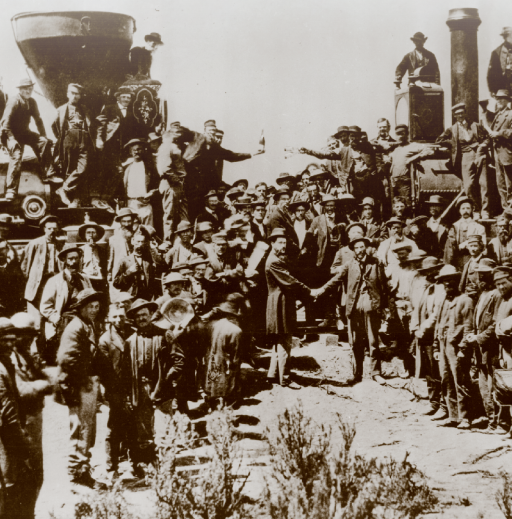
Workers joining the tracks for the first transcontinental railroad
